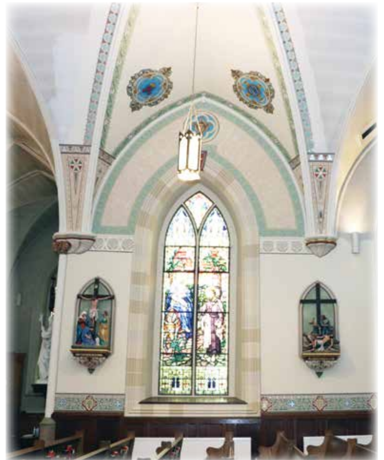
Here is a view of what the restoration will accomplish when the project is completed. The Stations of the Cross have been refurbished and the original frescoes have been replicated along with the trim.
