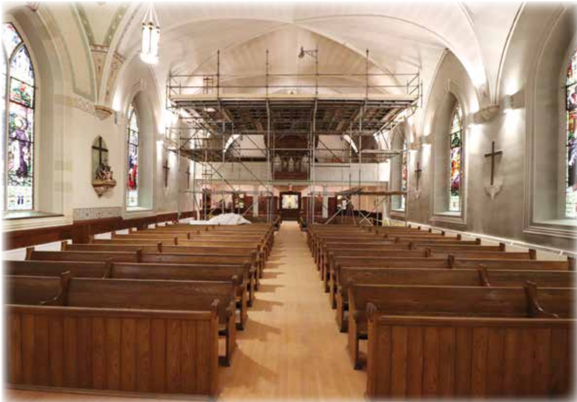
As the work on the ceiling continues the scaffolding will be rolled along allowing the artists to do their work. To accomplish this process pews must be removed as the work progresses.
