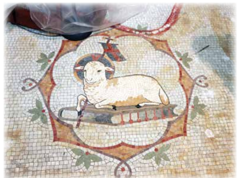
Here is a portion of the beautiful mosaic floor in the sanctuary. As you can see there is much work to be done in repairing and cleaning the floor.
